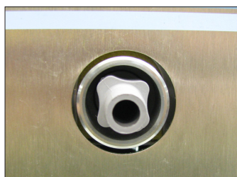
Installed Drain Fitting with Cap Removed
