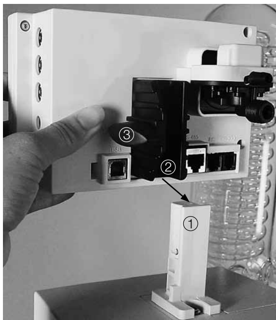
Fig. 5.12: Installing the vacuum controller
